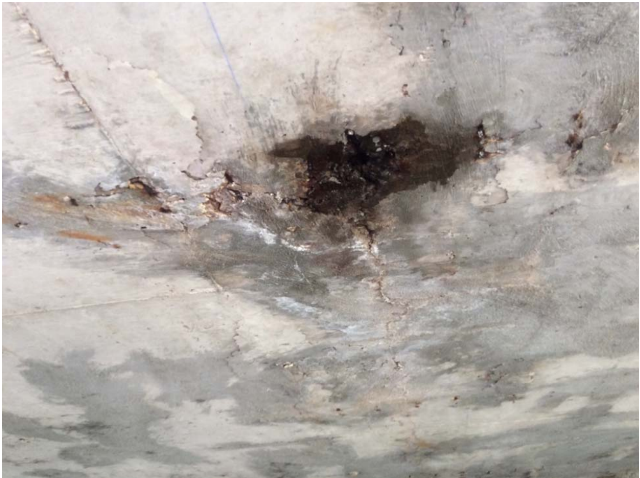
Span#3, spall at sonavoid drain
