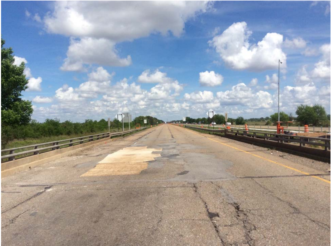
Note: 2 " ACHM overlay on bridge deck.
