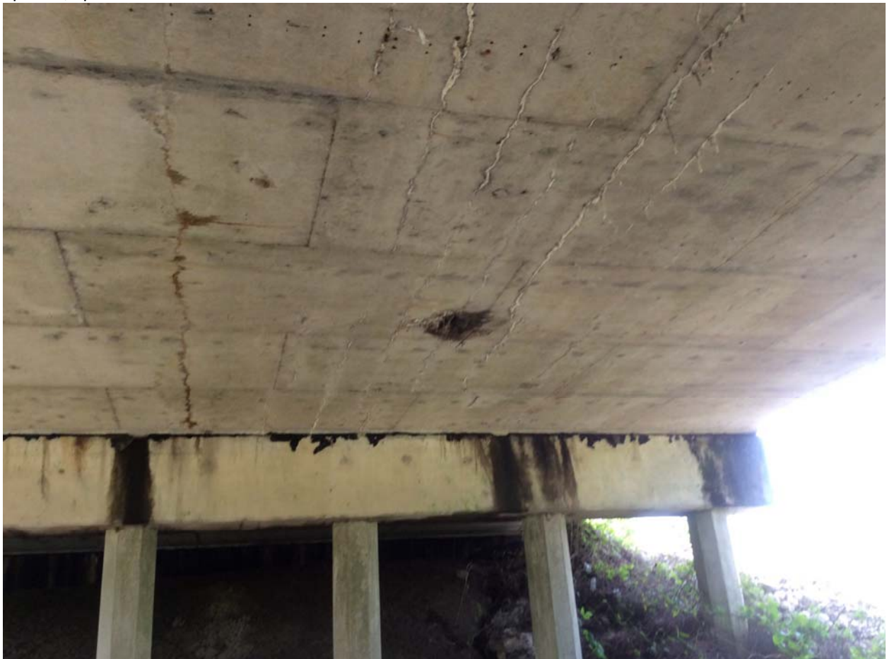
Span#3, spall at sonavoid drain
