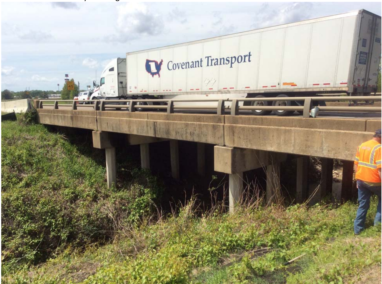
Note: 2 " ACHM overlay on bridge deck.
